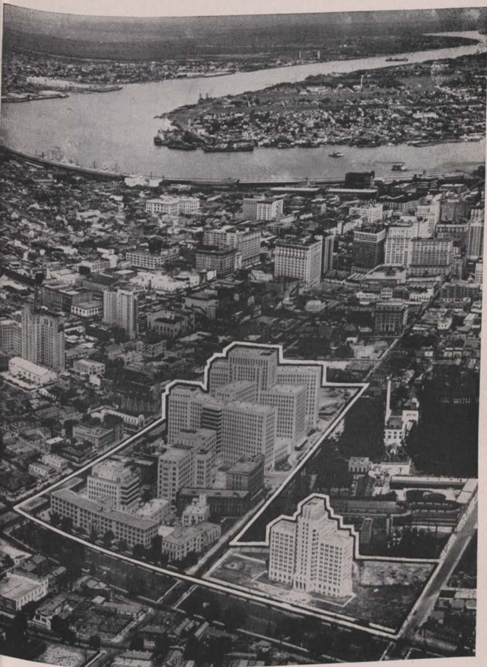
Aerial view of Charity Hospital Group (circled) made in 1940
